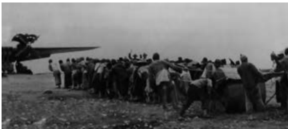
Chinese peasants at Yun-nan-i airfield pull a giant concrete roller in order to tamp down the landing strip's foundation.
