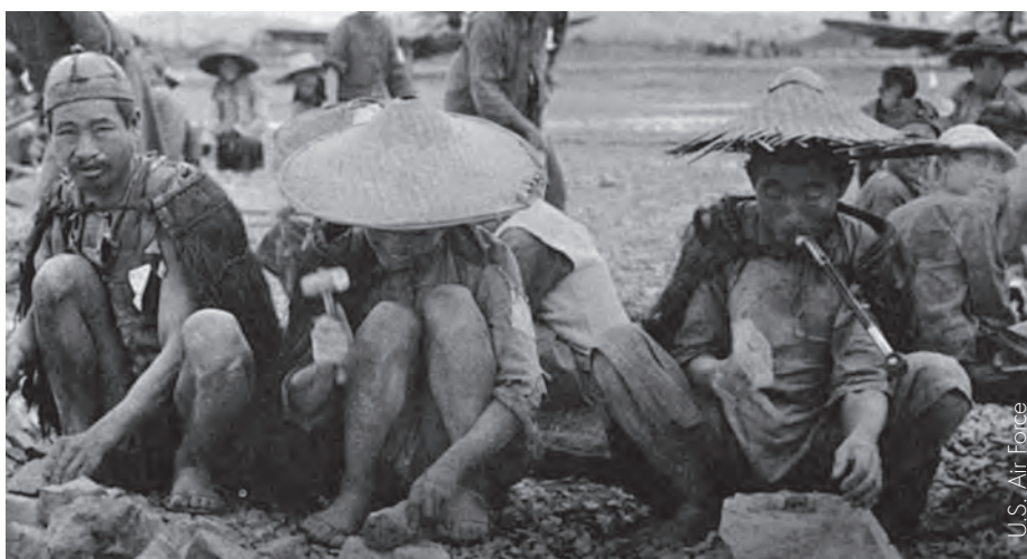
Chinese laborers breaking rocks into smaller pieces for use as gravel during airfield construction, c. 1943
