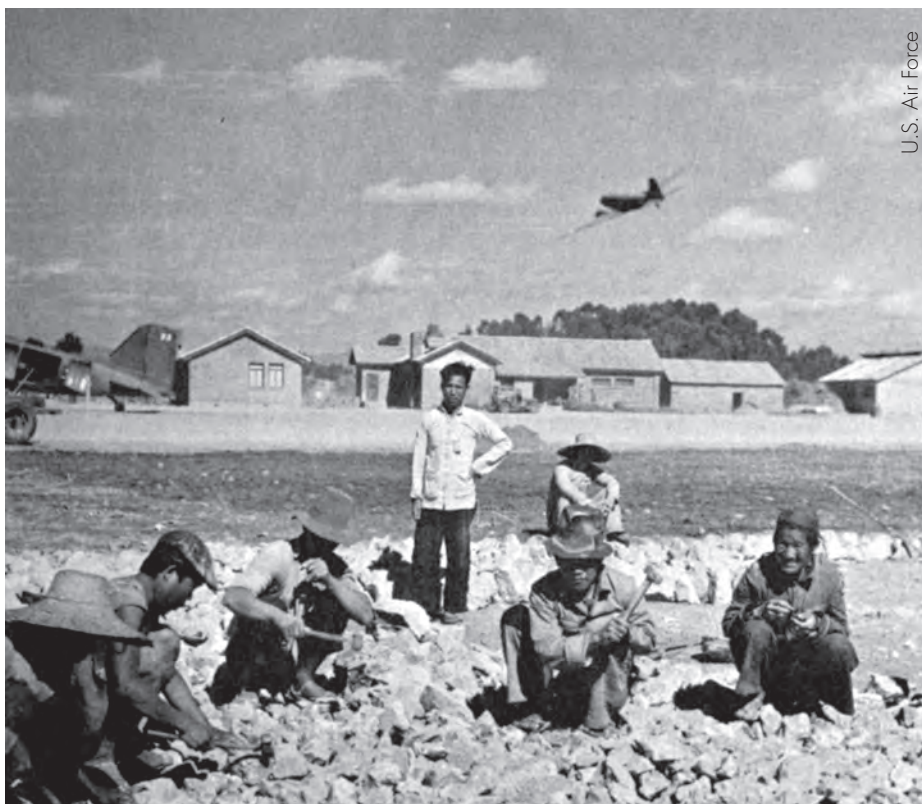
Workers breaking rocks to be used for airfield construction at Kunming, c. 1942
