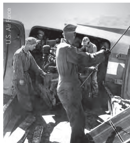
Army engineers unloading a partially disassembled bulldozer from an Allied transport plane, c. 1942
