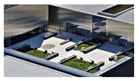
to add a sense of dynamism to the facade. Because the complex itself lies on a three-foot grid system, with every joint and edge of the building falling on these subdivisions with precision, each aluminum fin is spaced 18 inches apart to fall exactly on the edges of the laser-cut panels.
